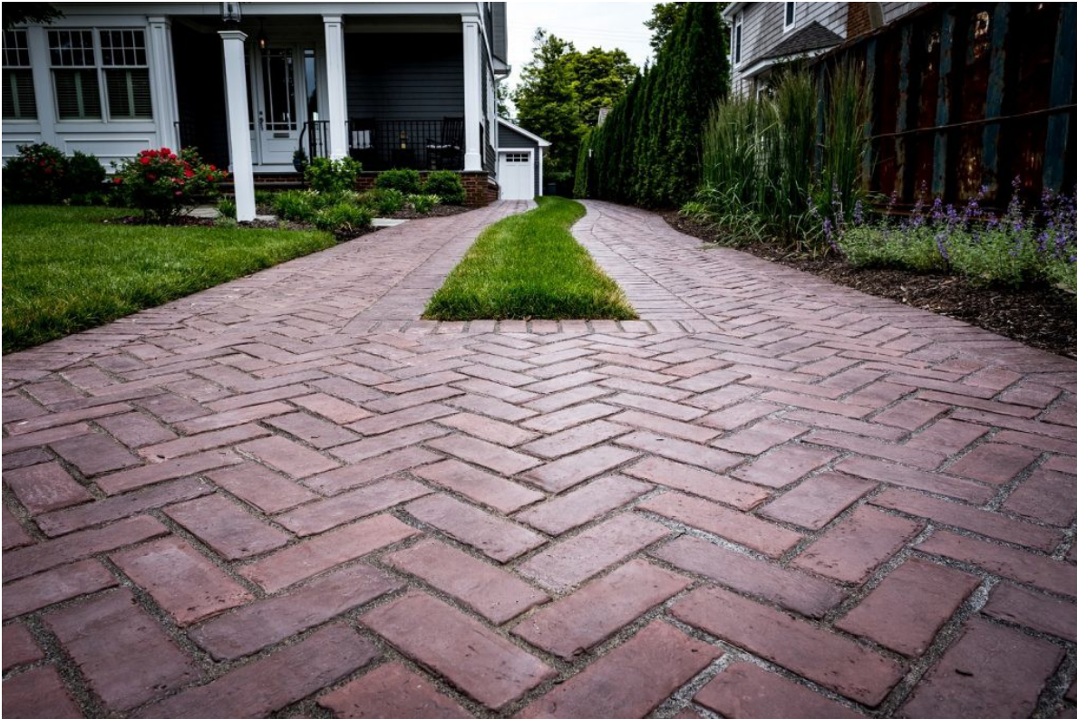
Figure 2: Ribbon Driveway with Pavers
